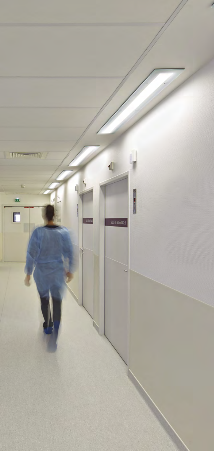
The range STAGNO is suitable for operating rooms or clean rooms.
